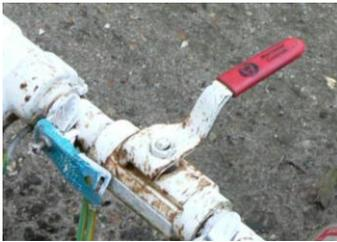
The outlet valve is often left open. If not, then turn on the outlet valve by rotating the lever to be in-line with the pipe.
