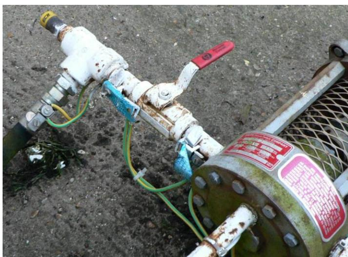
Fill the tank using the LPG compound controls as outlined elsewhere. When full, the noise from the pump will change abruptly as the gas flow stops when an internal valve shuts and the gauge on the vehicles tank will not go up any more.
